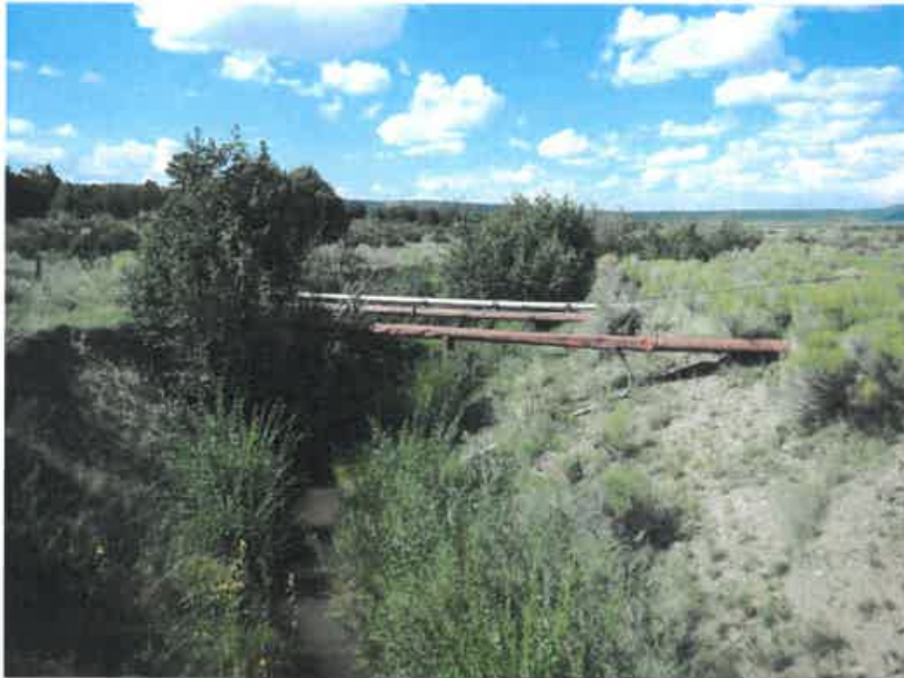
Photo 5-1: View of existing water infrastructure within the Parcel 1 Access and Utility Easement area
