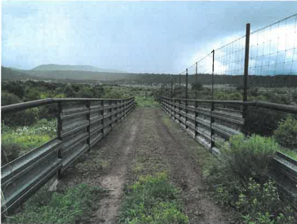
Photo 11-1: View of livestock/wildlife crossing bridge
